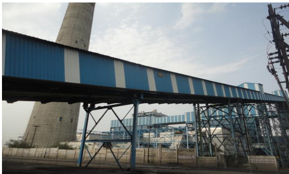
Closed type coal conveying system
